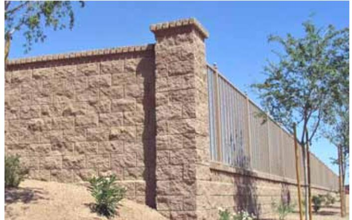
The 4" Proto-II™ Wall is also considered a "greener" product than the 6" or 8" masonry walls, using less concrete, cleaner steel, less masonry material and no grout. The use of less material contributes to the cost savings and efficiency of the system as well as the need for less labor and resources.
